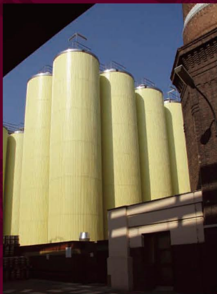
Conical-cylindrical tanks at the Staropramen Brewery in Prague
